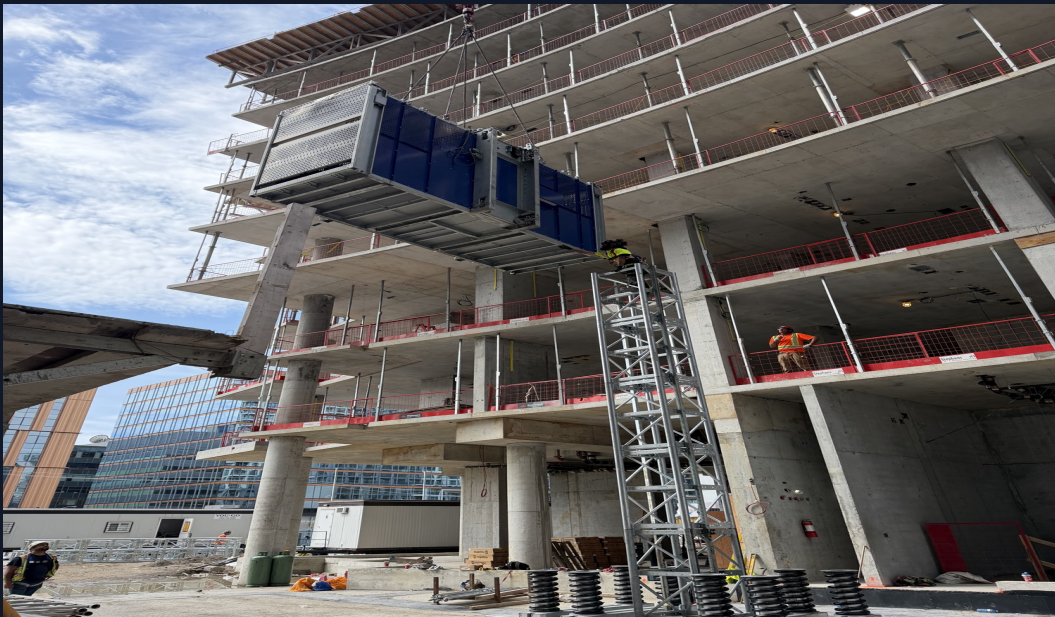
Crane-assisted equipment placement
