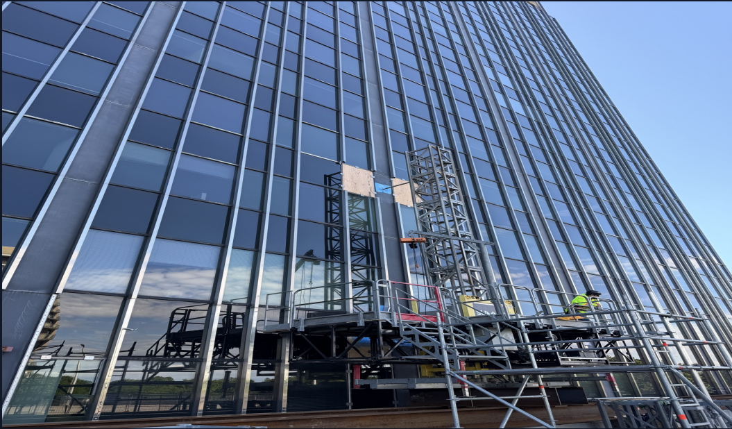
High-rise construction elevator install — GTA
